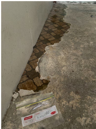
Photograph 9: Farmhouse 2 hallway floor to bathroom (friable asbestos detected)
