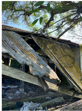
Photograph 12: Farmhouse 2 Dairy – collapsed roof area
